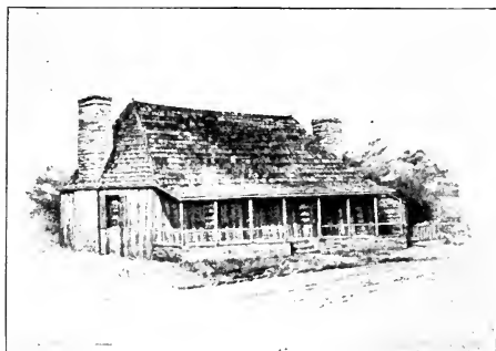
The Alexander McNair House, Property of the First Governor of Missouri.
